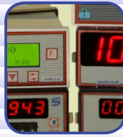
LEVEL CONTROL SENSORS
